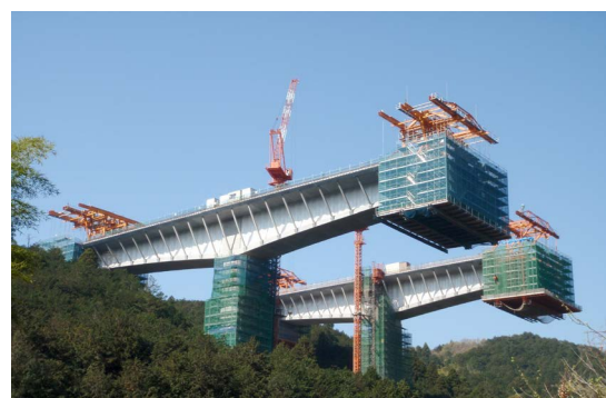
Fig. 2 Yatogawa Bridge under erection
