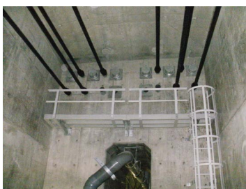
Fig. 9 Galvanized multi-PC cable
