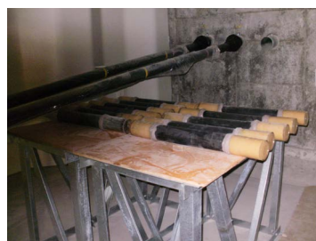
Fig. 10 Sample cables inside box girder
