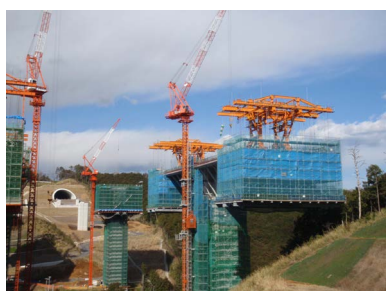
Fig. 13 Large-scale form traveler
