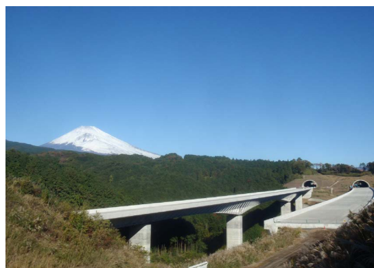
Fig. 1 Completed Yatogawa Bridge
