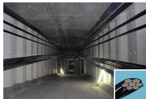
Fig. 8 Epoxy resin-coated PC cable
