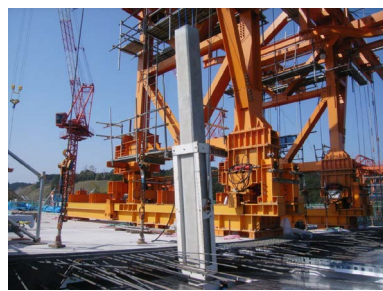
Fig. 14 Installation of RC struts
