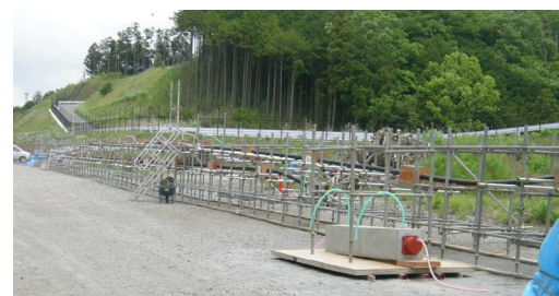
Fig. 11 Grout injection test
