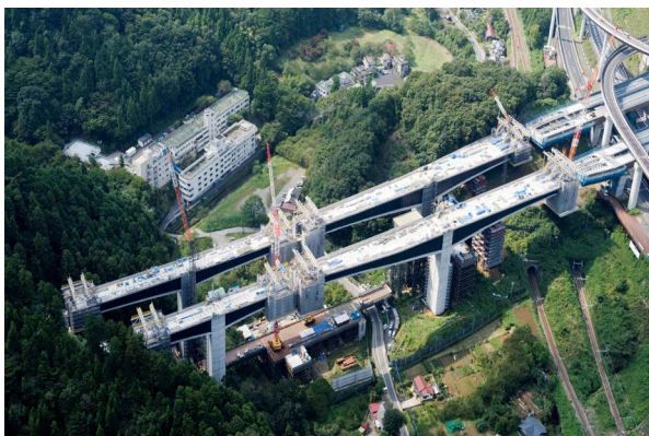
Fig. 4 Construction of superstructure
