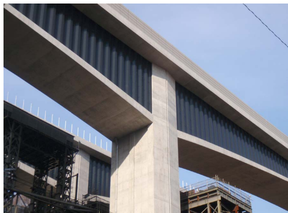
Fig. 7 Color of corrugated steel web and the bridge pier shape developed
