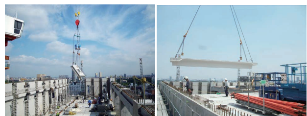
(a) Erecting PCa wall panels
