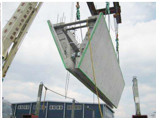
Fig.10 Conditions of suspended members
