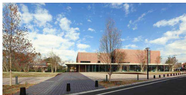
Fig.1 Outside view of the building
