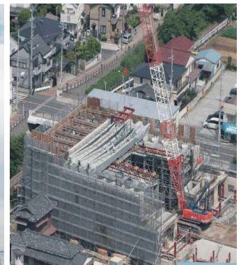
Fig.11 Conditions of erection
