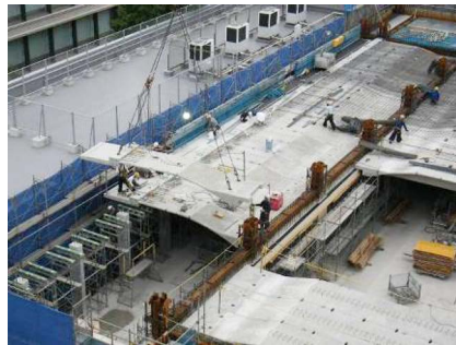
Fig. 12 Placement of PCaPC slabs (PS3)
