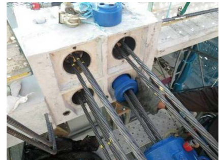
Fig. 13 Tension end of PCaPC slabs (PS3)
