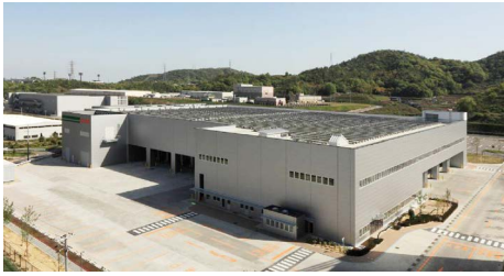
Photo. 2 External view of Stage 2 building
