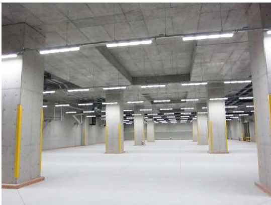
Photo. 3 PC flat-beam girder
