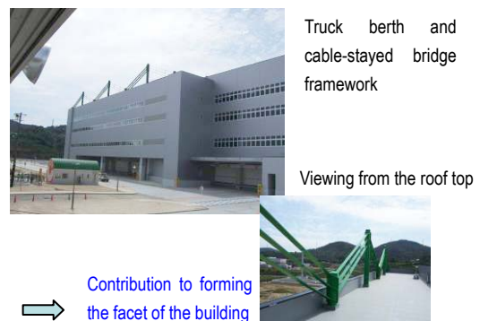
Photo. 7 Truck berth of Stage 1
