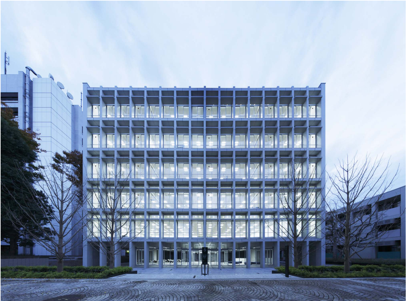
Fig.2 Latticed-pattern facade of the New 5th Building
