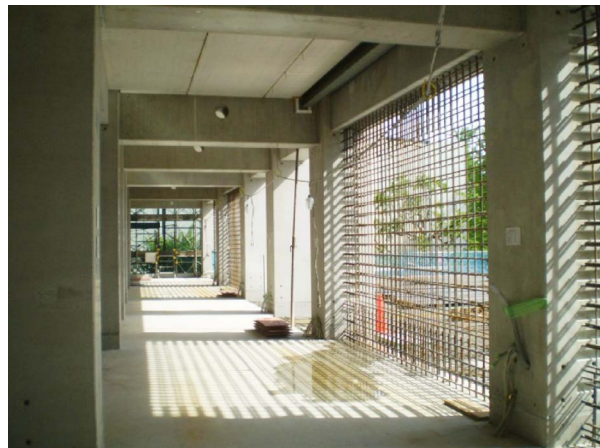
Fig.12 Reinforcing bar arrangement of bearing walls
