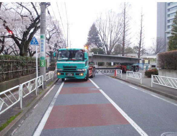
Fig.10 Transportation of ST slabs
