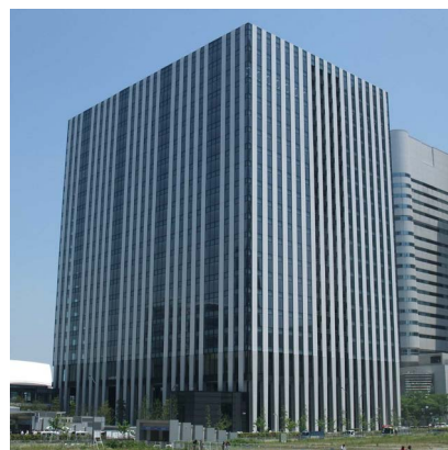
Fig.1 Minato Mirai Center Building
