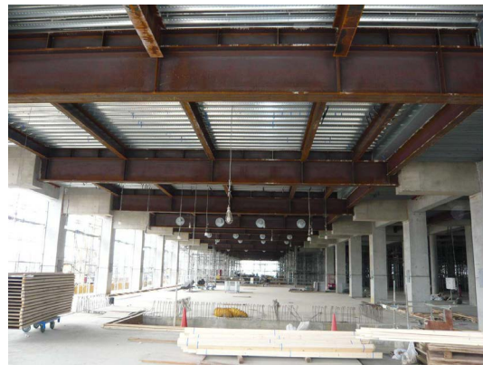
Fig.6 Hybrid composite beam (under construction)
