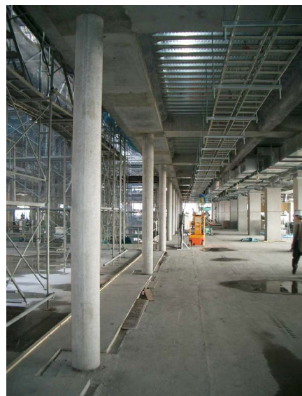
Fig.7 Slender precast column (under construction)
