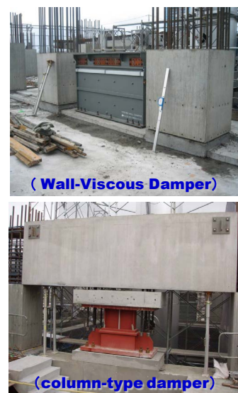
Fig.10 Installation of vibration control devices
